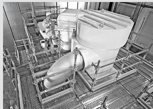
Working scaffolds industry
