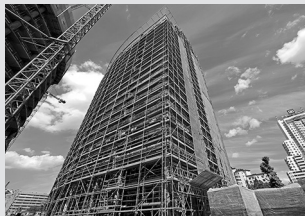
Working scaffolds facade
