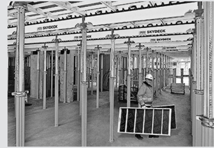
Slab formwork
