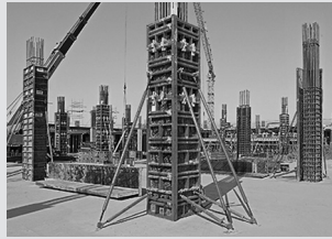
Column formwork
