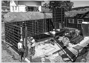
Wall formwork
