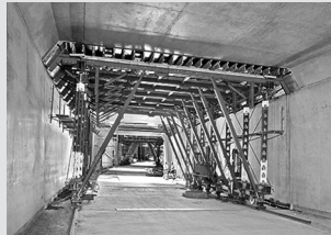
Tunnel formwork
