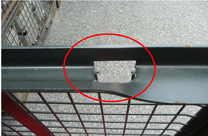
32.06 Deformed crane eye
